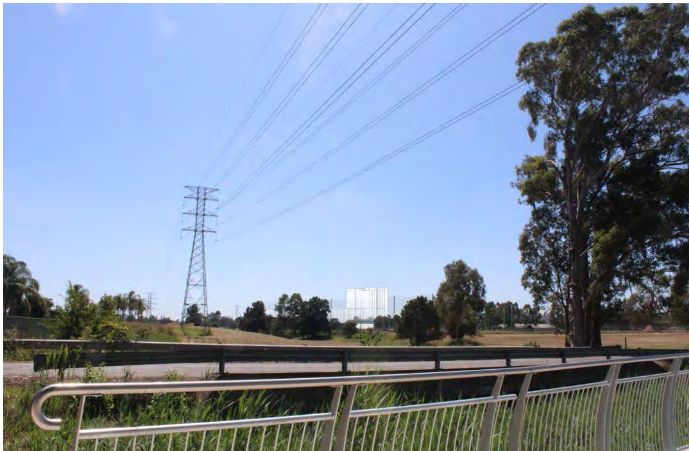
View 06 View from Jamison Road looking towards the southern boundary of the site. 14 storey building is visible from this location whilst the existing vegetation screens the smaller scale buildings.
